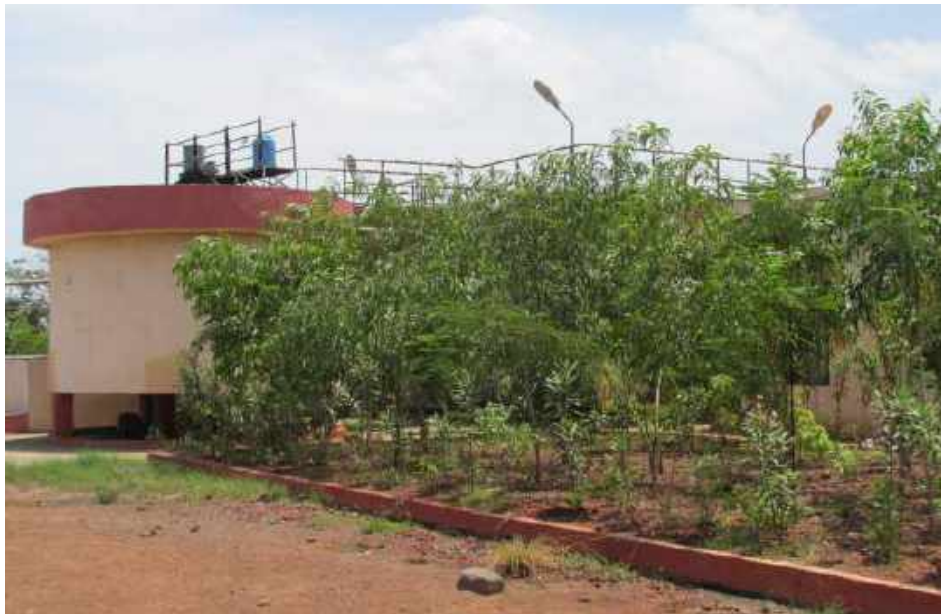
Fig. 1.5: Sewage Treatment Plant (STP)
