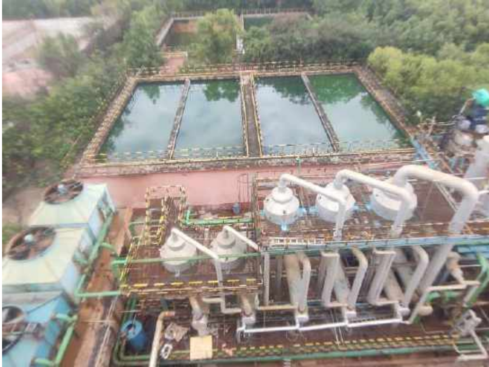
Fig. 1.10: Guard ponds for storage of treated Effluent
