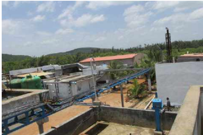
Fig. 1.3: Desalination plant in the Hetero Premises
