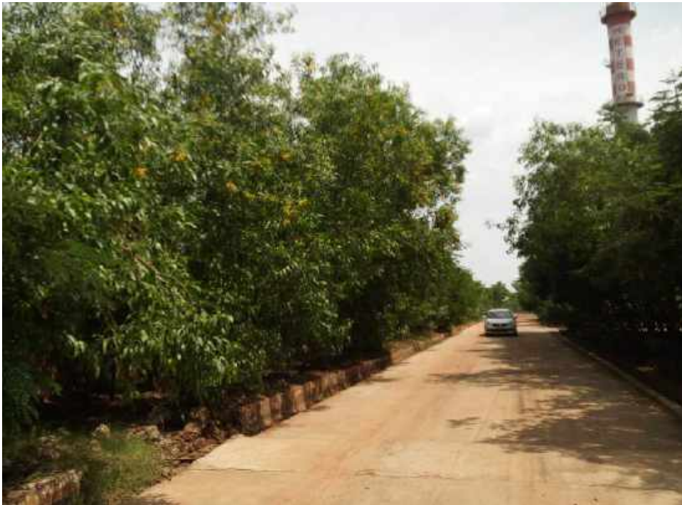
Fig. 1.15: RCC Road connected to Boilers with Green Belt
