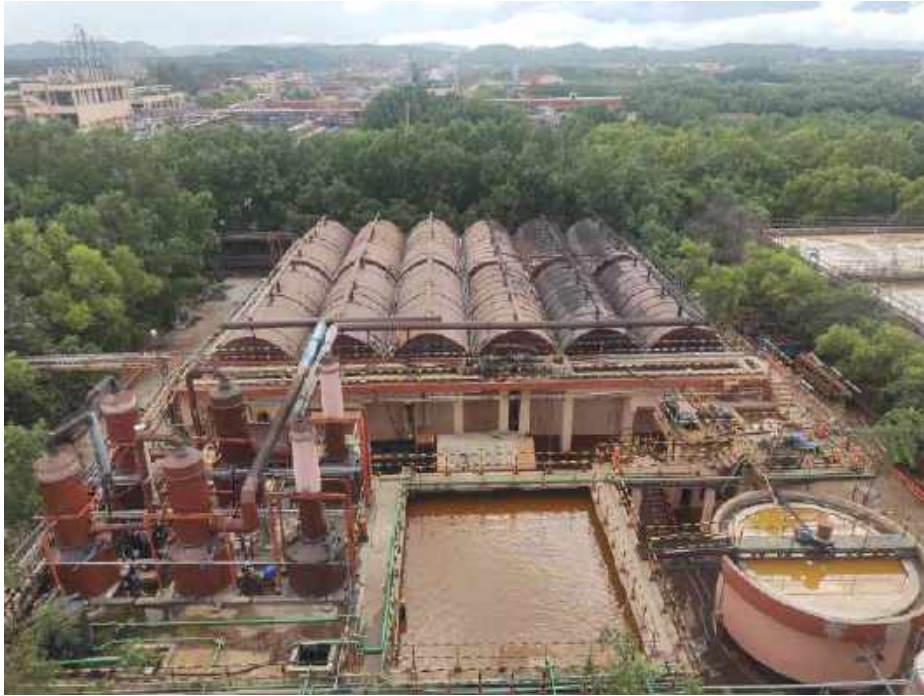
Fig. 1.8: HTDS Tanks covered with Hoods and connected to Scrubbers
